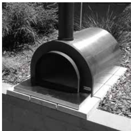
(Sitting the oven on top of a concrete on bricks and blocks)
