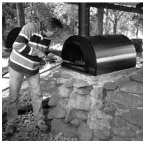
(Sitting the oven on top of a concrete on bricks and blocks)
